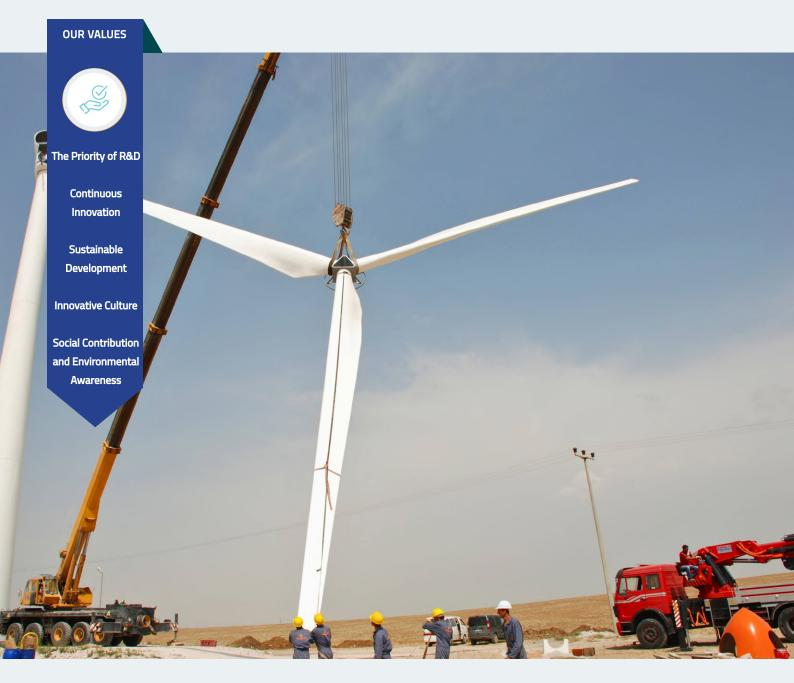
The production, optimization, and installation of Türkiye's first unlicensed 250 kW wind turbine have been completed. With the SoyutWind brand, production of residential wind turbines has begun to meet the 2006 clean energy needs of homes.
