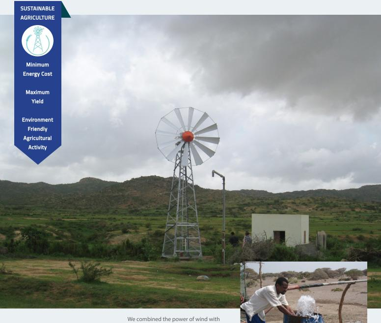
We combined the power of wind with water in Africa with the Soyut WindMill wind water pump, which was produced and exported with 100% in-house design and engineering (2009).
